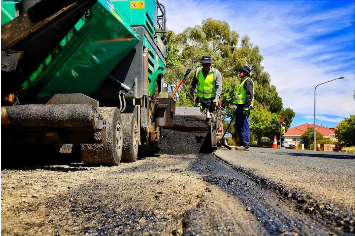
Asphalt is a mixture of sand, aggregates such as gravel, and bitumen. (ABC News: Greg Nelson)
